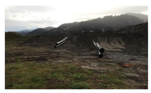
Upper photo shows piping through embankment, lashed to floats on ends inside the basin. The pipe on the left is an overflow pipe, and the one on the right is the segment connecting to the "spreader pipe. The photo below shows the overflow and spreader pipes. The spreader is laid along the hill contour, with its end elevated, available for cleanout if necessary.
